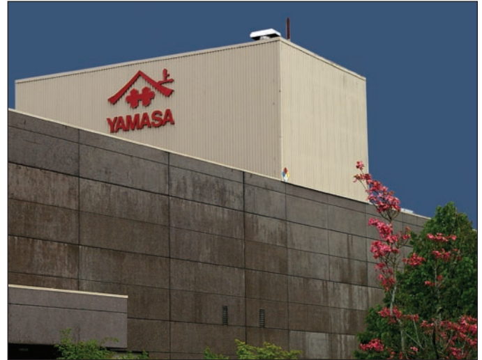
Yamasa facility on Fairview Industrial Drive in South Salem.
